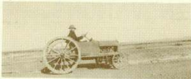
Tractor made from Overland car, made by Cliff and Ron Gibb.
